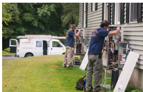
PICTURE 5B-2. INSTALLATION OF RESIDENTIAL HEAT PUMPS
