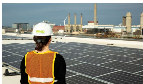
PICTURE 4-1. WORKER ON SOLAR ROOF ATOP THE WIND TECHNOLOGY TESTING CENTER
